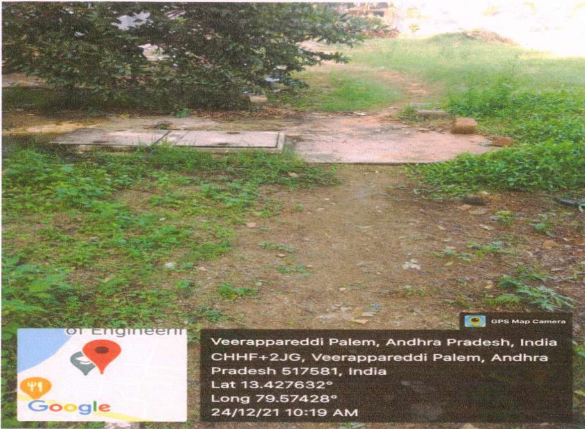
Closed drainage – liquid waste storage
