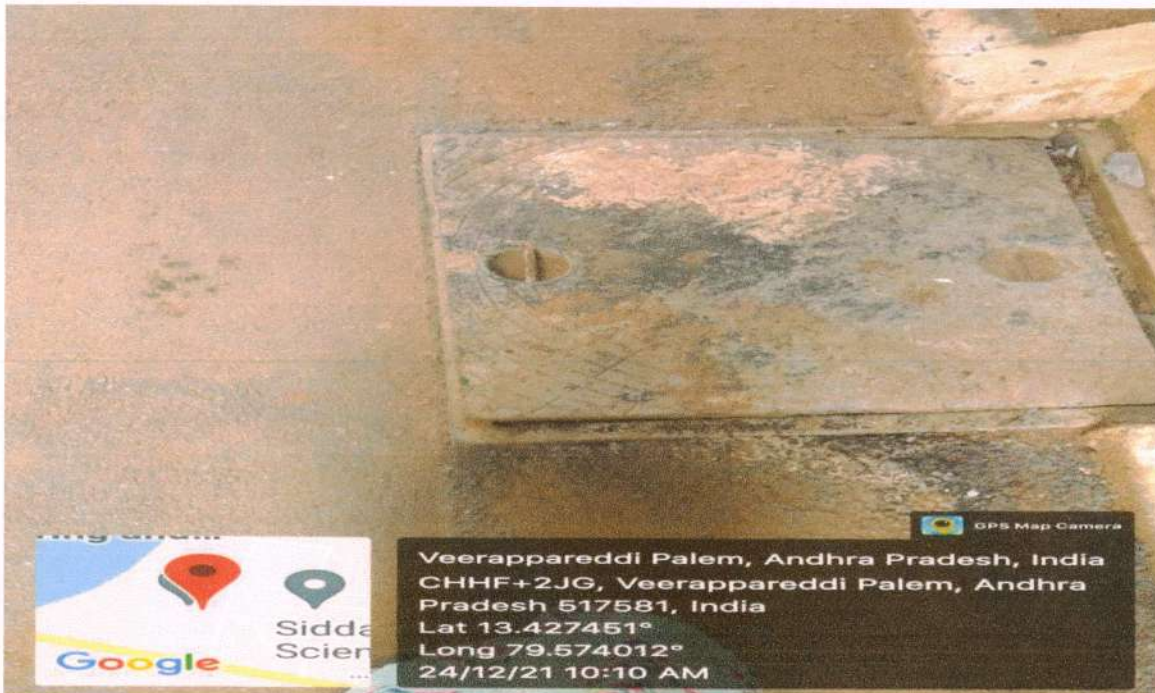
Closed drainage – collecting liquid waste
