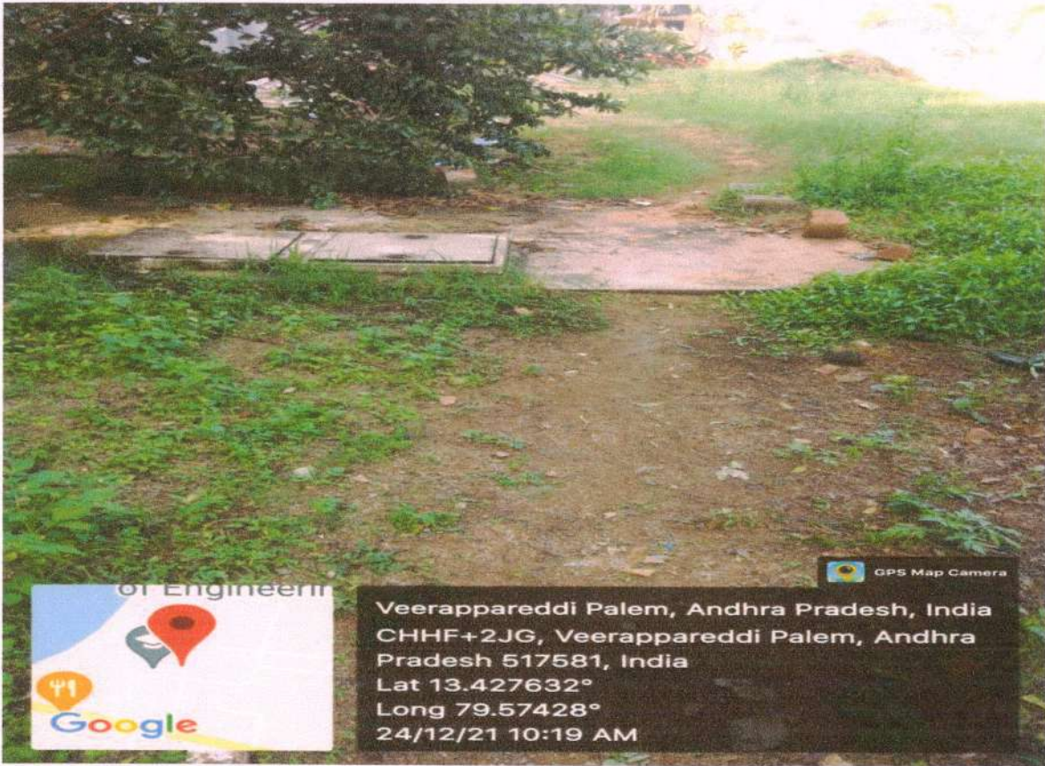
Closed drainage – liquid waste storage
