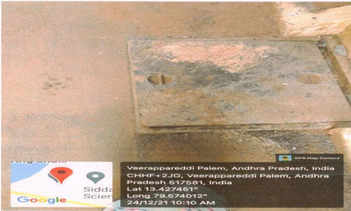
Closed drainage – collecting liquid waste
