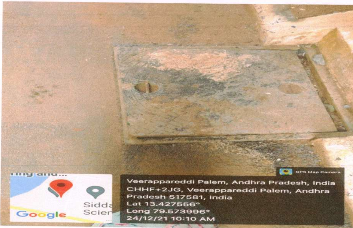
Closed drainage – collecting liquid waste
