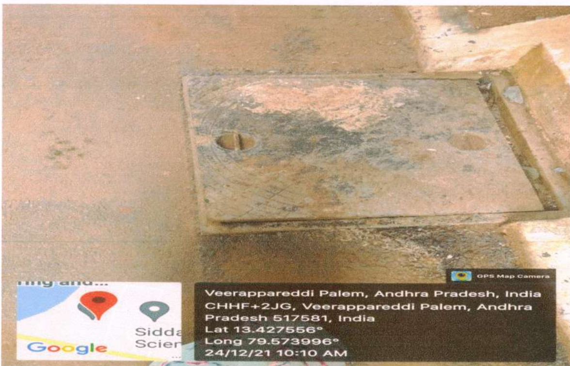
Closed drainage – collecting liquid waste
