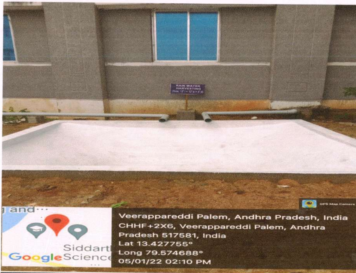
Collecting rain water through closed pipes
