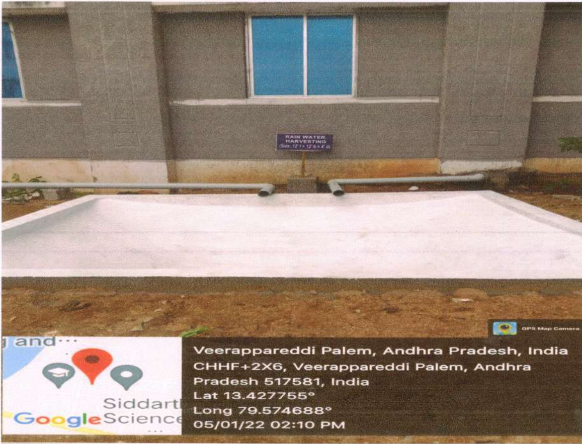
Collecting rain water through closed pipes and rainwater harvesting pit
